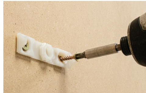
9 Attach the WISKA® COMBI® 308 bracket to the wall
