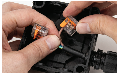
6 Attach connectors onto floodlight wiring
